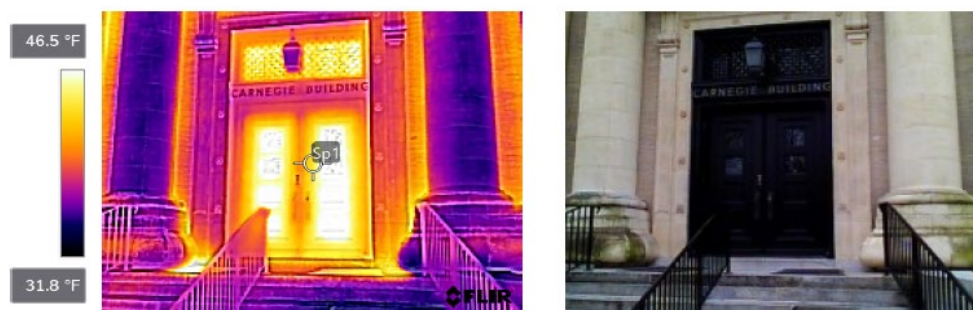
Figure 12: Infrared Image of the Main Entrance Doors
