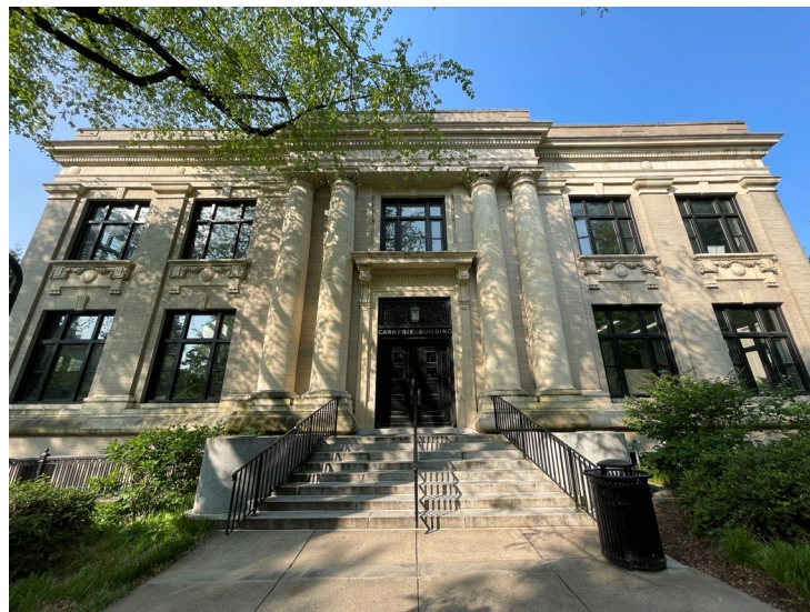
Figure 1: Main Entrance of Carnegie Building
